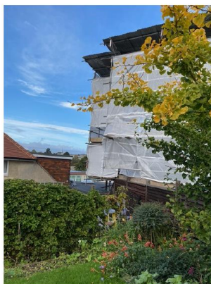
Fig. 1: view from 112 Denton Drive during the work
