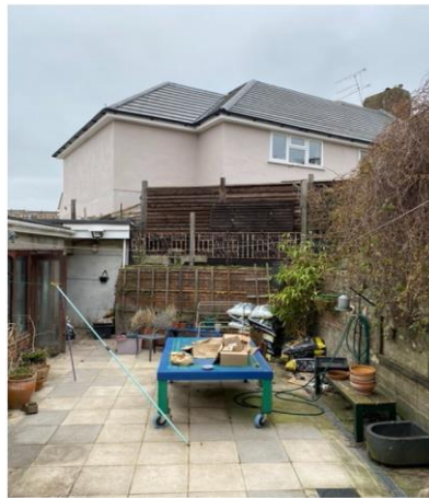
Fig 2: view of development at 10 County Oak Avenue from 112 Denton Drive
